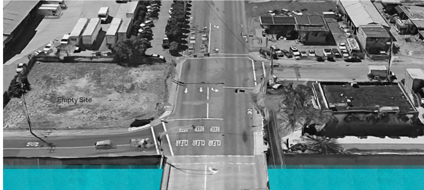
Existing storm water pipe below Spurce St
