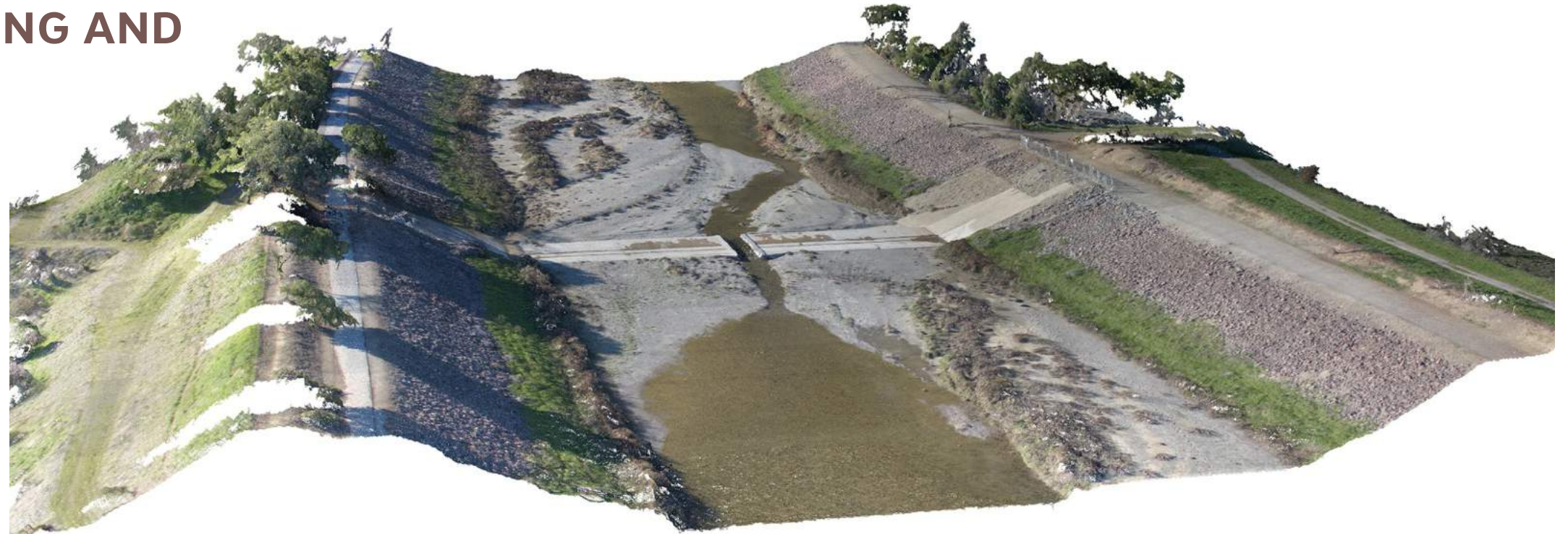
PHOTGRAMMETRY MODEL OF NOTCHED FOUNDATION OF FORMER RUBBER DAM #2 (CHANNEL STATION 50,000); SURVEYED ON JANUARY 28TH, 2018
