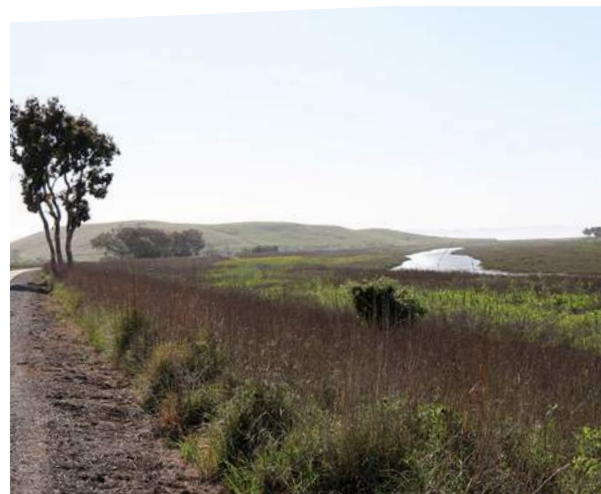
ALAMEDA CREEK FLOOD CONTROL CHANNEL
